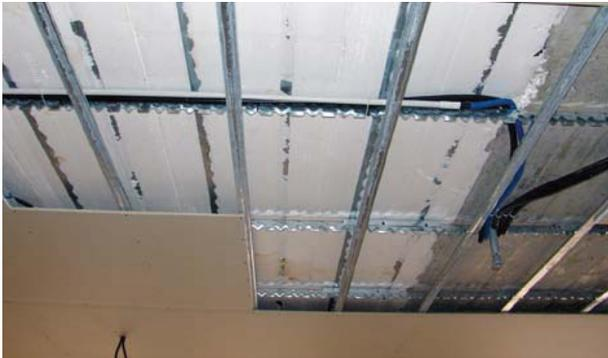
**Model C** - for internal dry finishing with built-in metallic profiles exposed with interaxis 30 cm - panels are not fitted with any metal grid as they are meant to be left raw or covered with gips boards, false ceilings or any kind of internal dry finishing.
