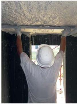
**Model I** - for internal plaster finishing with plaster-holder mesh installed; panels shall be coated at the intrados with a stretched, hot-dip galvanized metal grid as a plaster support, incorporated to the panel to avoid thermal bridges.
