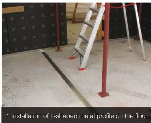
1 Installation of L-shaped metal profile on the floor
