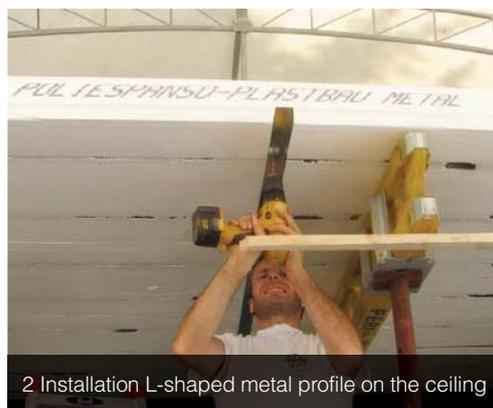
2 Installation L-shaped metal profile on the ceiling
