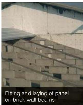
Fitting and laying of panel on brick-wall beams
